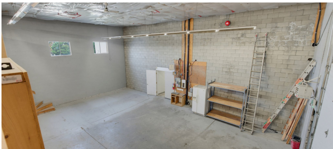
SHOP AREA — OVERHEAD DOOR, BLOCK WALLS, SERVICE PANEL
