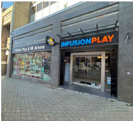
YATES STREET FACADE
